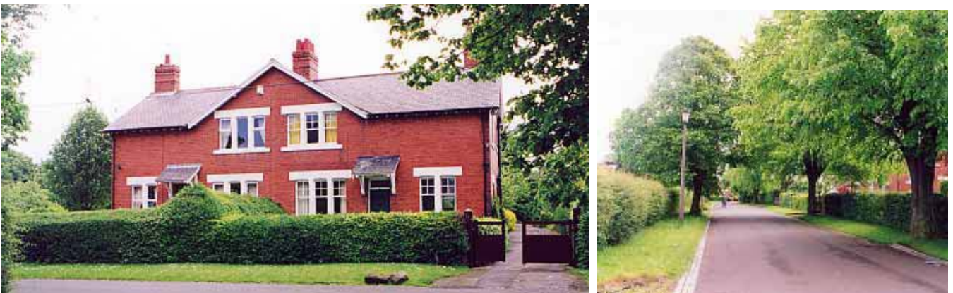
Above left: numbers 14 and 16 Northumberland Gardens, typical of the house type and setting of this sub-area. Above right: view along unadopted Northumberland Gardens.
